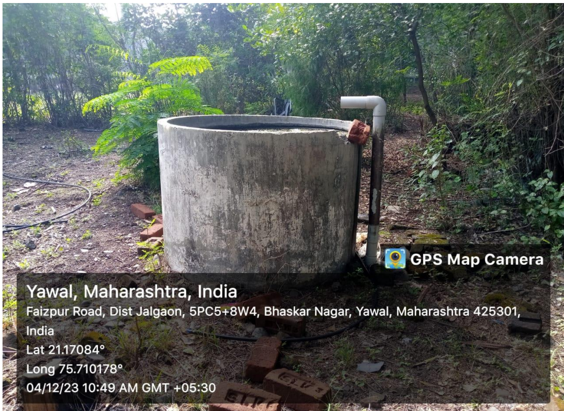
Water Tank in Botanical Garden
